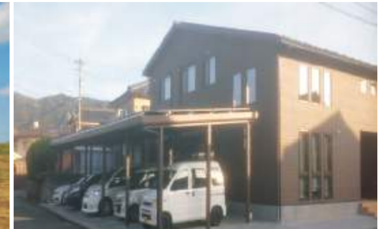
50kw carport solution in Japan
