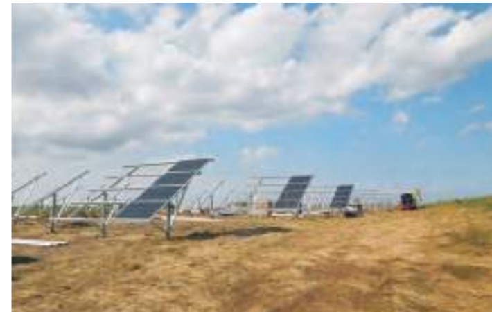
760kw pile ground solution in Holland
