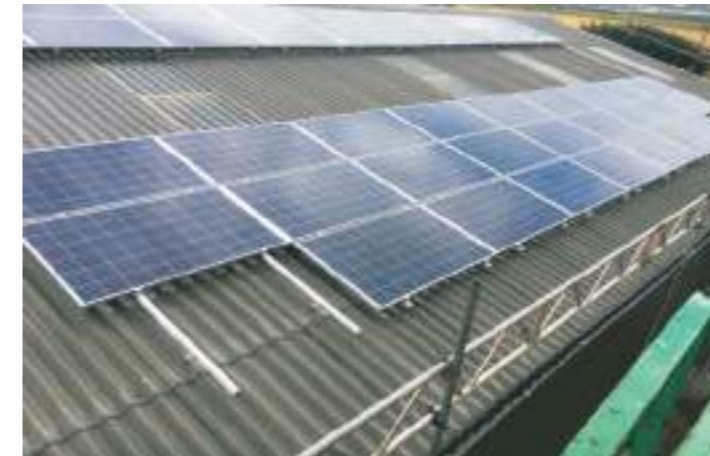
105kw hanger bolt solution in UK
