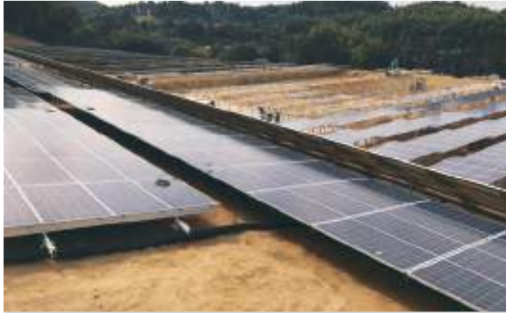
2.0mw ground screw solution in Japan
