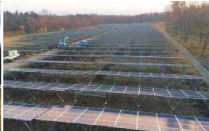
4.3mw ground screw solution in Japan
